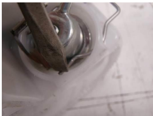
Photo 7: In some cases it may be necessary to push down on the end of the retaining wire ends to align them to the holes/slots in the module body. Take care to keep the ground wire under the retaining wire.
